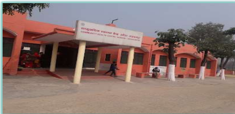
A Primary Health Care Center in Saharanpur District
